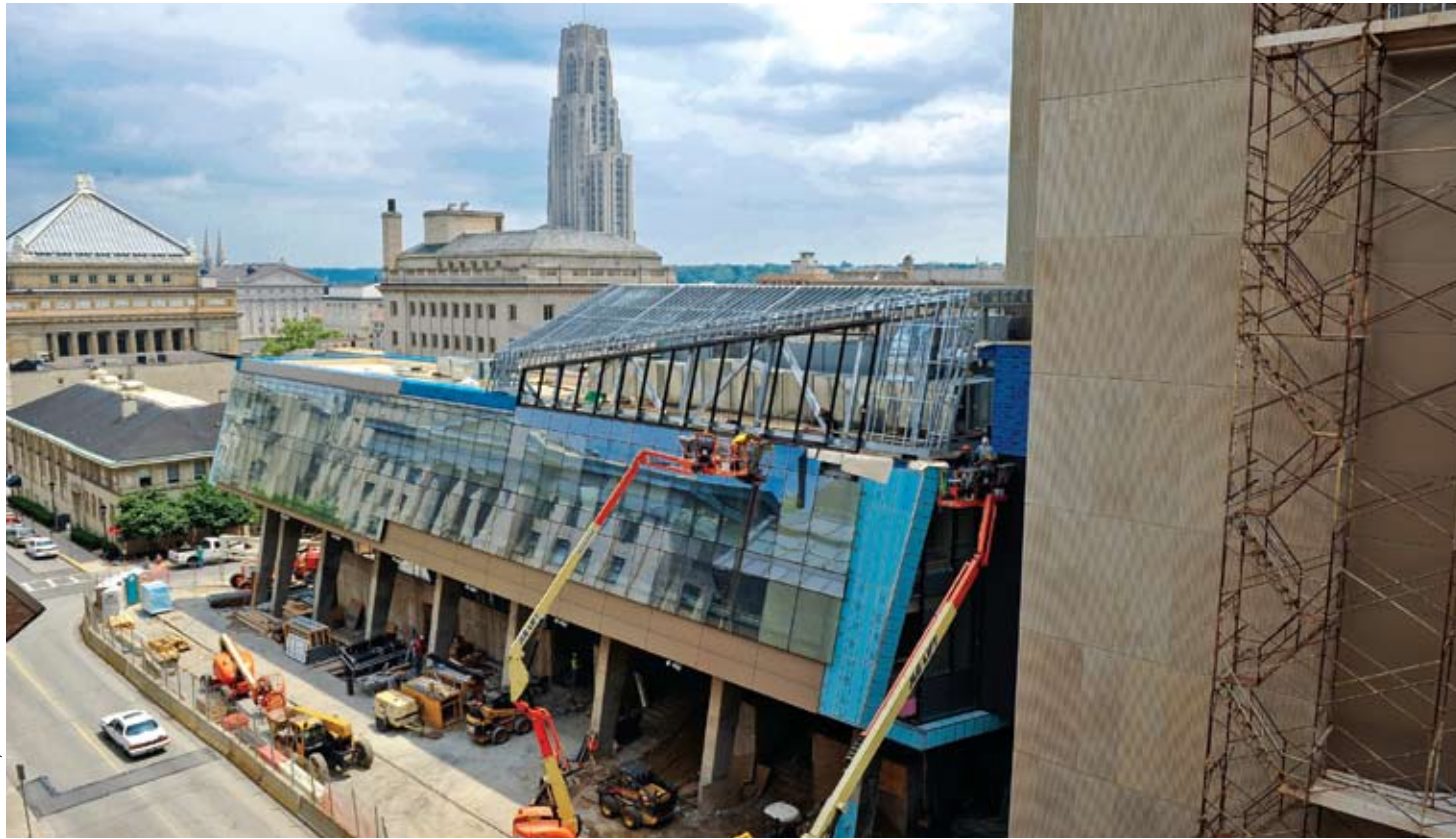
The Mascaro Center of Benedum Hall under construction
