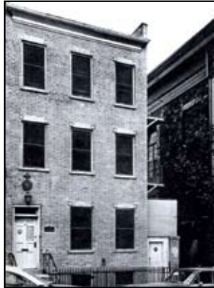
House at 2 Oliver Street, New York, 1821. Connoisseurship methodology allowed Toker to attribute this modest house to the obscure architect James O’Donnell.
