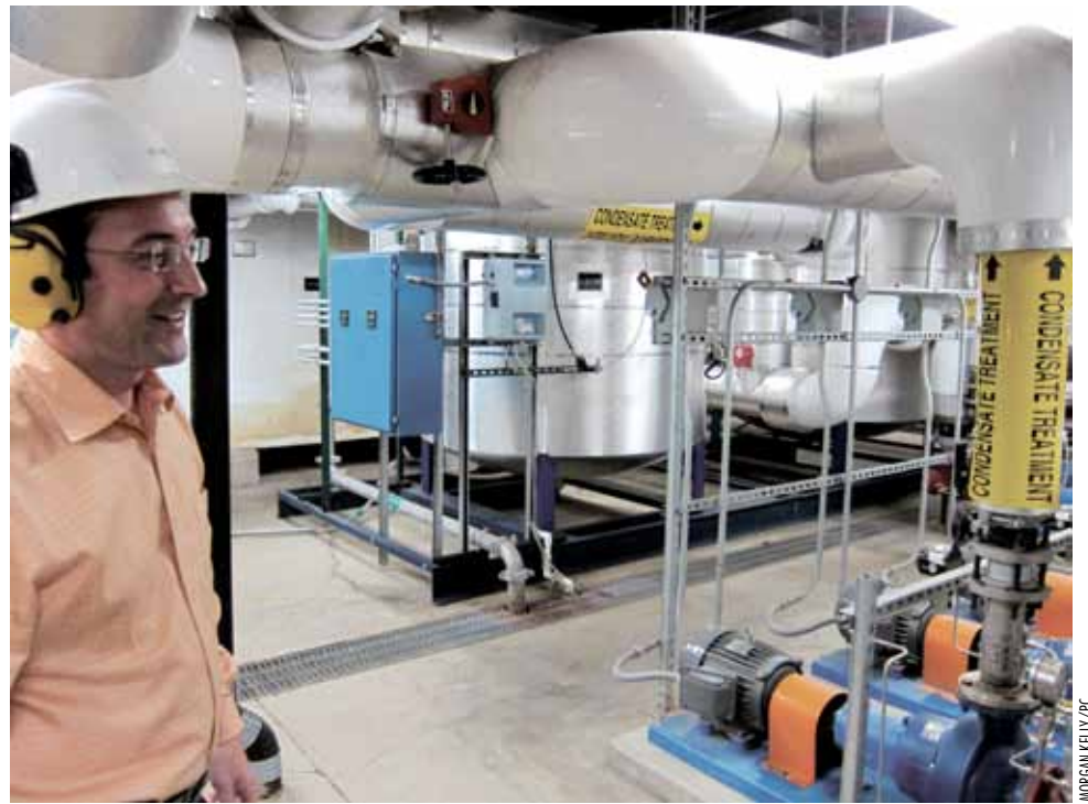
Above: Carrillo Street Steam Plant manager Marian Gagu stands before rows of industrial purifiers that monitor and control the pH balance of water heading into the boilers.
