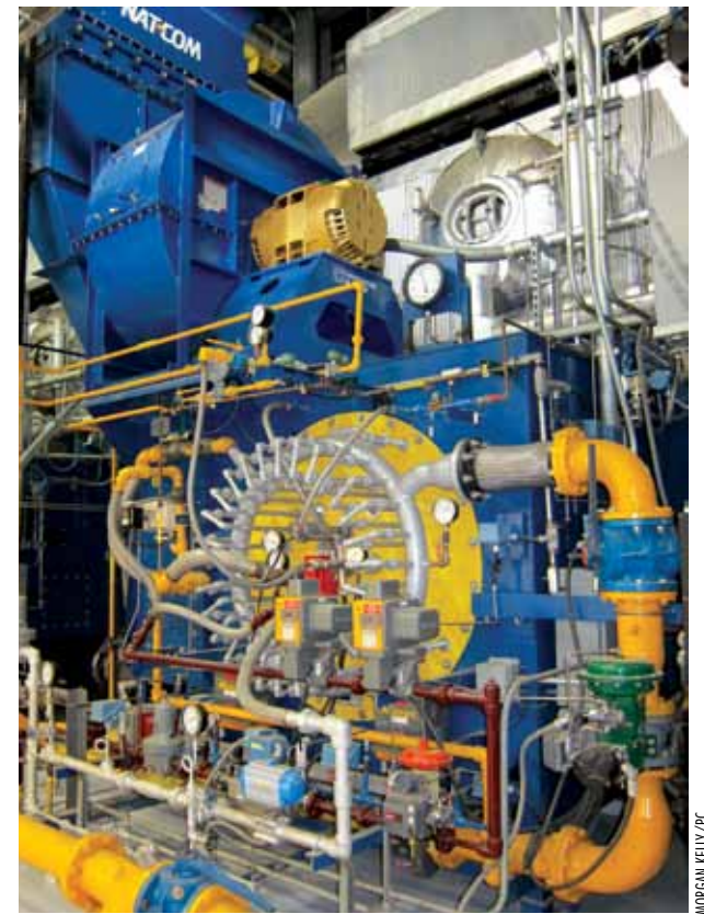
Each of the six massive Carrillo Street boilers transforms roughly 14,000 gallons of water per hour into 115,000 pounds of steam.
