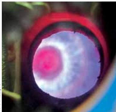
A large spiral-shaped flame keeps the internal temperature of each boiler within the toasty range of 1,200 to 1,300 degrees Fahrenheit.
