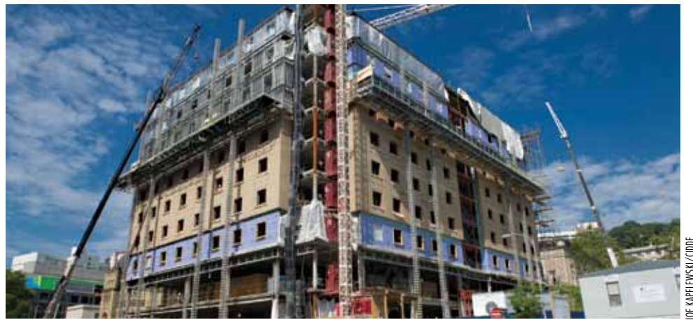
New freshman housing being built on Fifth Avenue will include a health services center.
